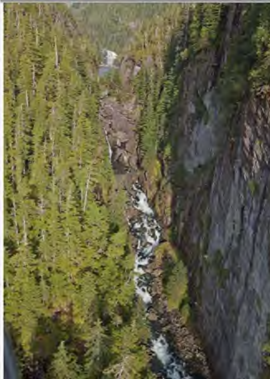
Photo 3-1. Leakage Flows from Falls Lake through the Colluvium Outlet
