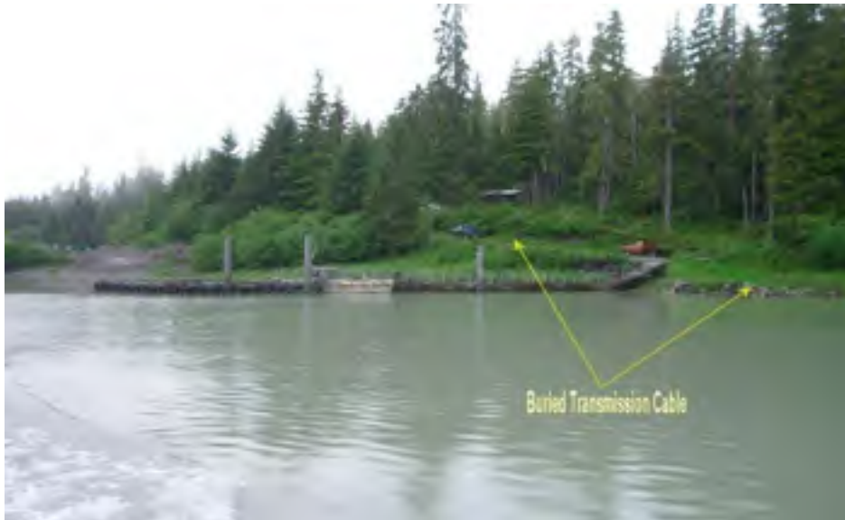
Photo 3-30. Transmission Line Landing at Existing USFS Dock in Thomas Bay.
