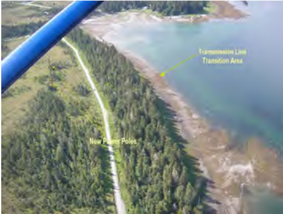
Photo 3-31. Frederick Sound Shoreline Cable Connection
